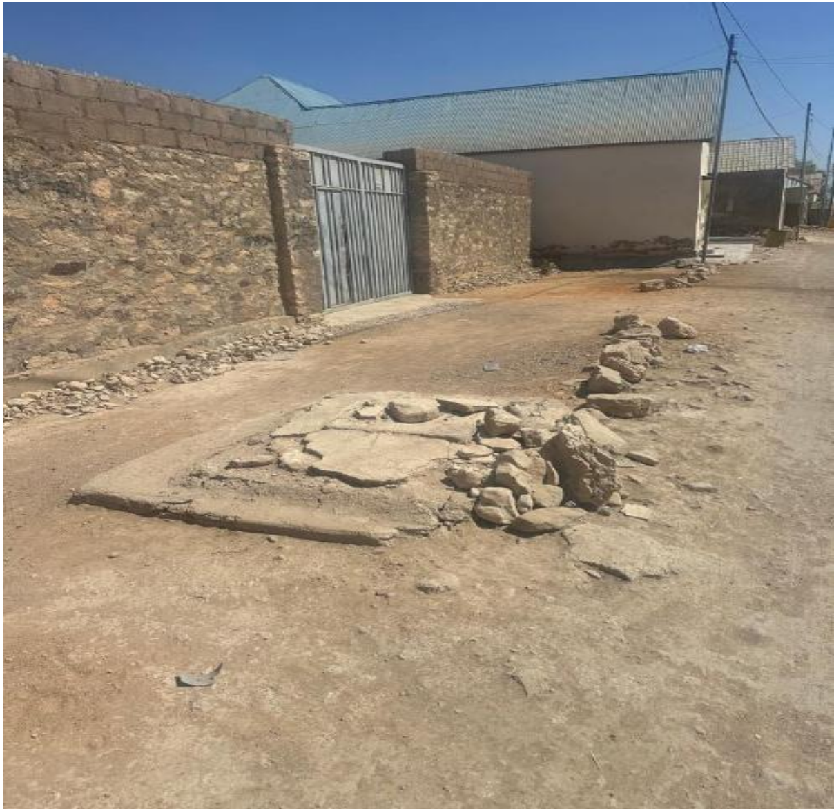
Figure 3: Shows an abandoned shallow well, no longer in use, situated within the right-of-way
